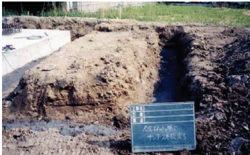
Laying SAN-EARTH M5C *One 25kg bag of M5C will cover approx. 3 meters (width 50cm) .
